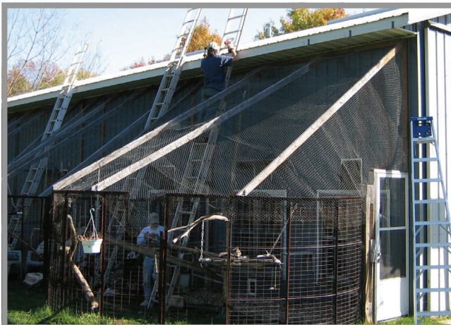
Some of our intrepid volunteers install new gutters.
